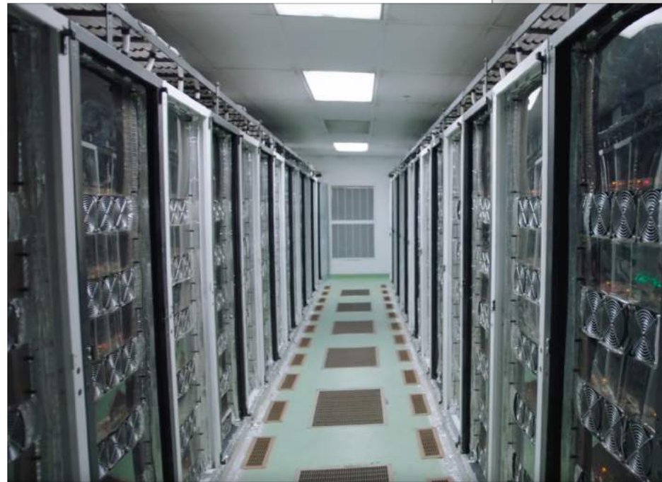
Hot Aisle/Cold Aisle Design
