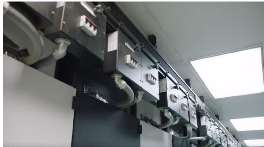
Overhead Power Distribution
