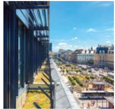
Bureaux Galeries Lafayette Rennes (35)
