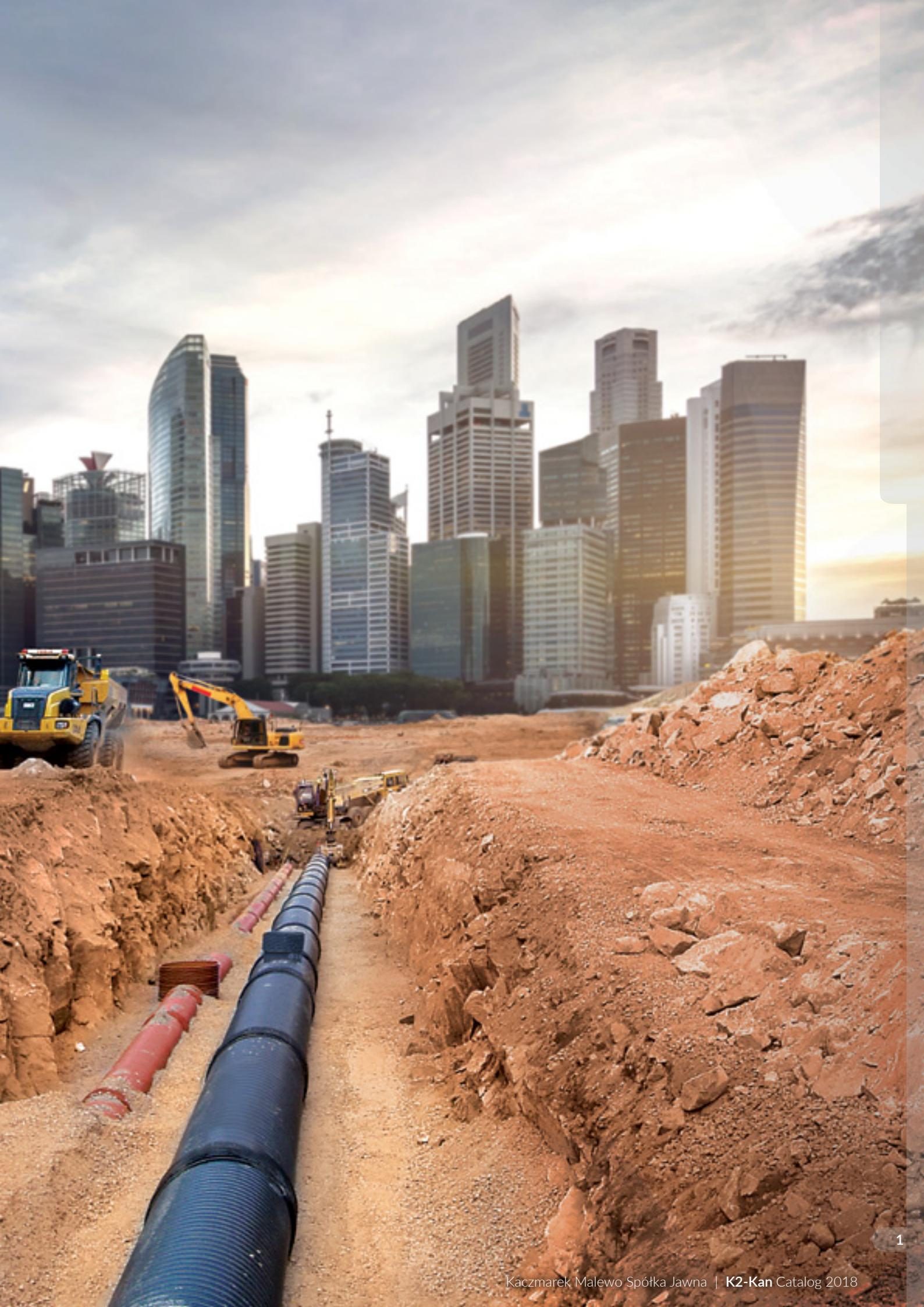
The K2-Kan system of polypropylene (PP) structured double-wall pipes for sewers. Searching for optimum solutions in construction of gravitational buried sewers and taking into account current works trends in production of plastic pipes, we have launched PP structured double-wall pipes and fittings that meet high technical requirements and are truly the **21st century** products.
