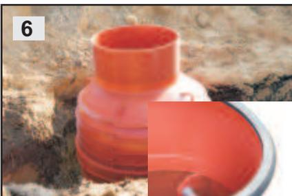
6 A taper should be installed similarly to other manhole components (rings  $\varnothing 1000$ ). A cylindrical section of the taper (from the minimum of 1 to the maximum of 25 cm) may be cut to achieve the required manhole height.
