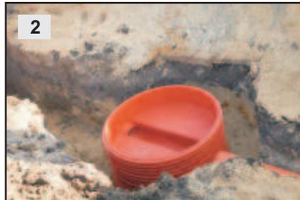
2 Place a base unit on a prepared earlier sand bedding and level it and then connect sewage pipes to the chamber. A place where a manhole is located should be lowered by approximately 10 cm. Connect sewage pipes.
