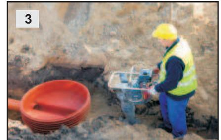
3 Fill up the trench with preliminary backfill (10 cm above the pipe level). Compaction should be performed manually, in layers every 15 cm or with light mechanical equipment (each layer up to 30 cm). Base unit 1000 should protrude above the backfill level.
