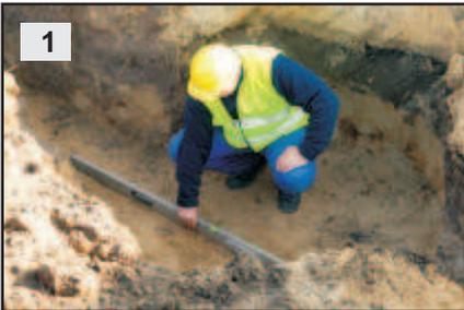
1 Prepare a trench in an inspection chamber location removing large and sharp-edged stones. On the trench bottom prepare bedding composed of compactable soil, preferably sand (coarse- medium- or fine-grained) of minimum 10 cm thickness. An inspection chamber zone should include an area of at least a 30 cm wide strip around the chamber.
