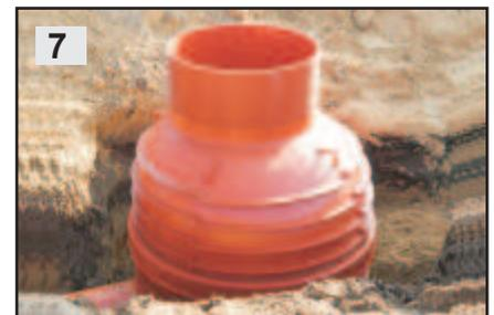
7 For shallow installations, taper 1000/600 may be connected directly to a base unit with no ring used.
