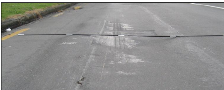
Membrane seal ‘bleeding’ through thin asphalt surfacing. Note line of ‘blooms’
