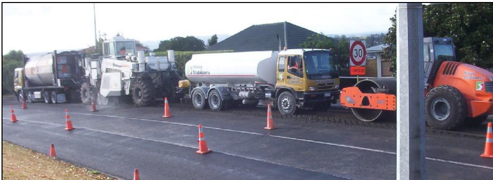
FBS in urban setting with an existing central concrete strip that was retained.
