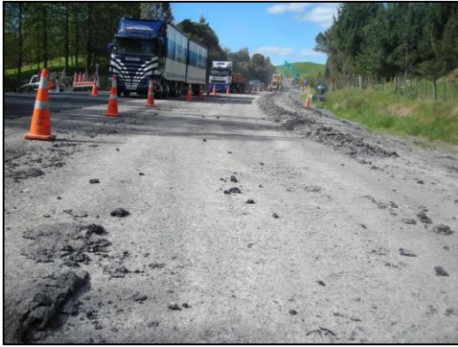
Removal of all seal
