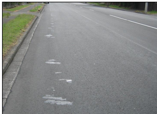
Membrane seal ‘bleeding’ through thin asphalt surfacing. Note line of ‘blooms’
