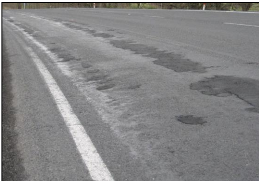
June '07 Primary wheel track repairs
