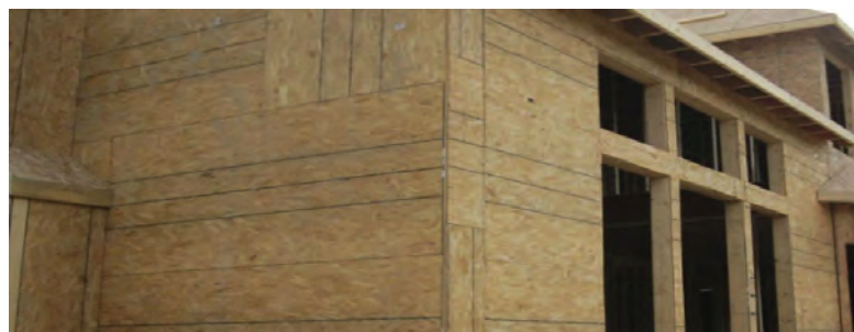
OSB as exterior wall sheathing
