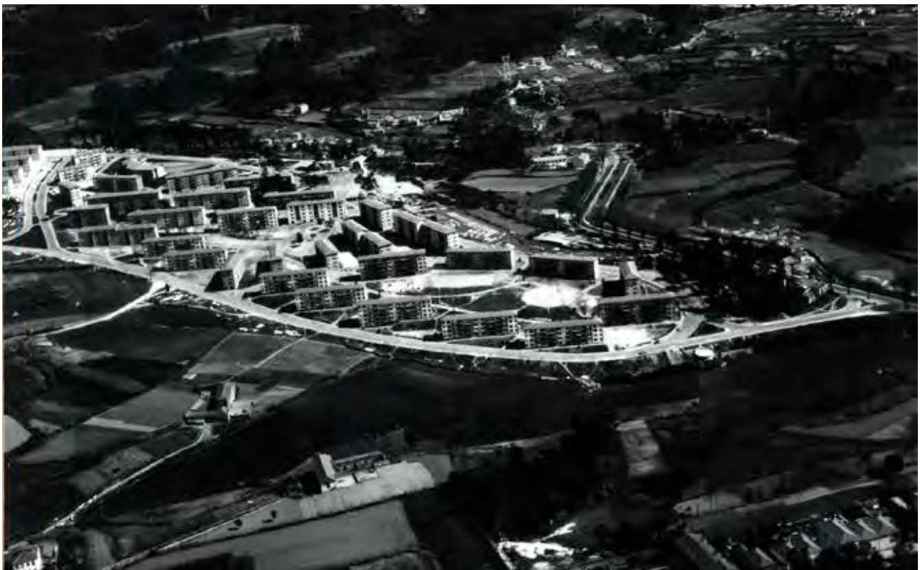
Figure 2. Cerco do Porto neighbourhood, 1961. Credits: Porto Municipality Historic Archive
