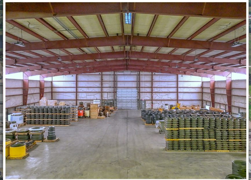
BUILDING A INTERIOR
