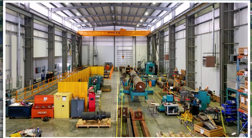
BUILDING D INTERIOR
