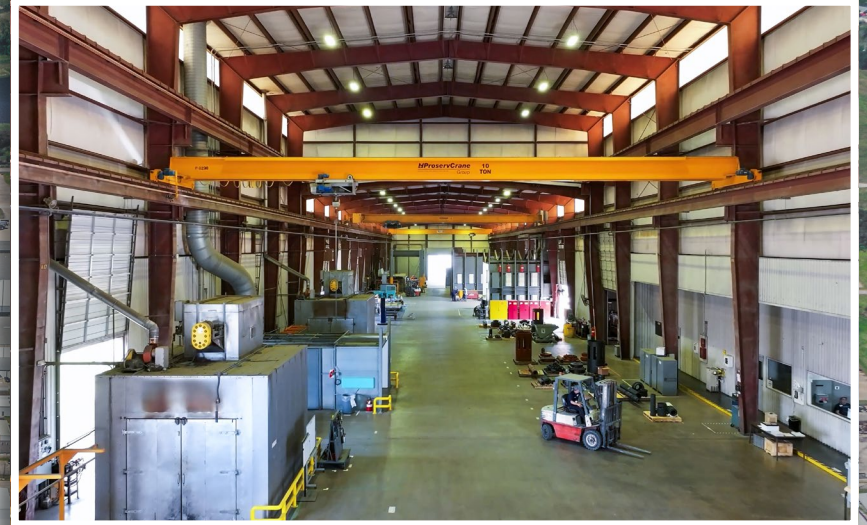
BUILDING E INTERIOR
