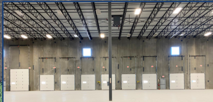
DOCK DOOR EXPANSION COMPLETE
