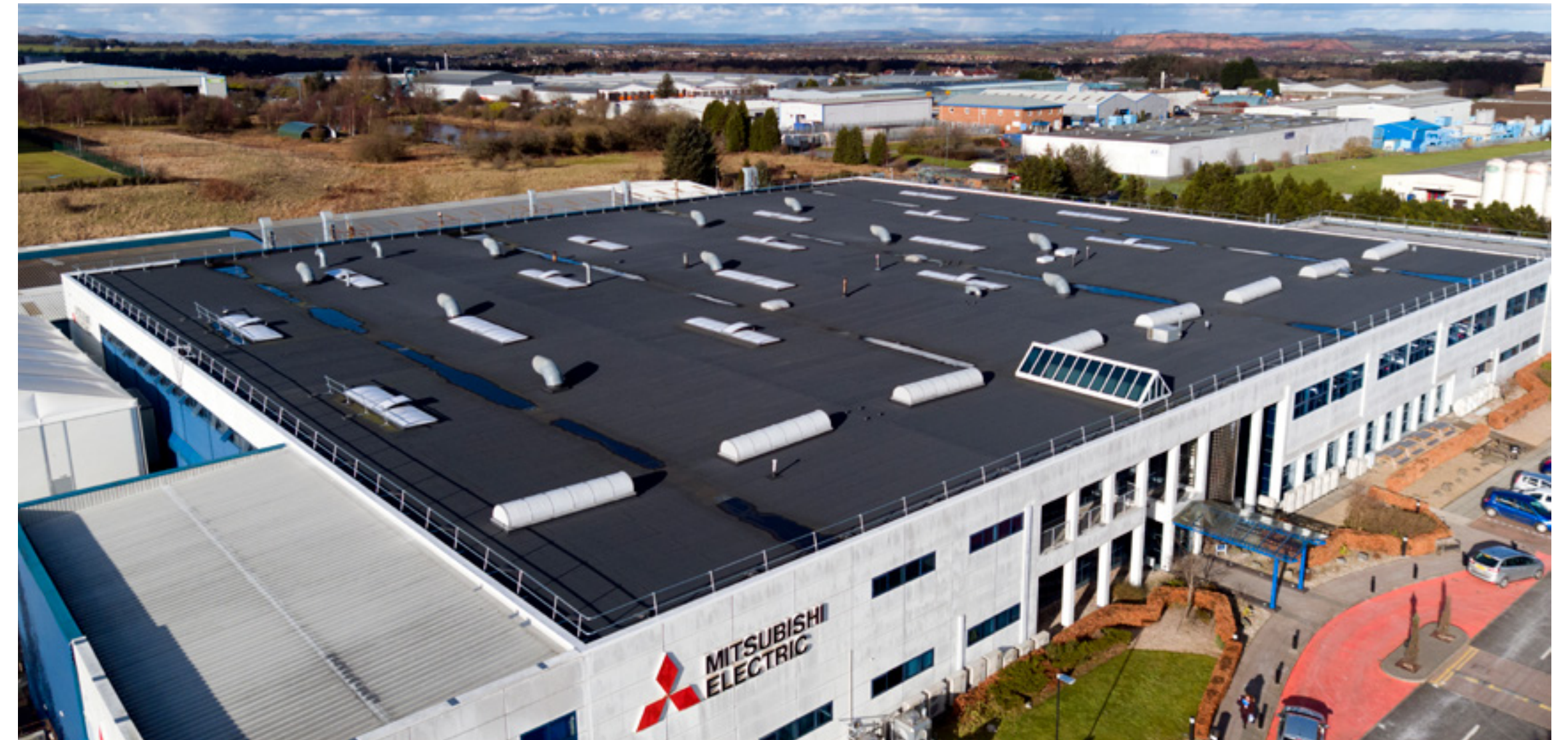
Mitsubishi Electric factory, West Lothian: BMI Icopal Thermosolo roof system (advanced SBS bitumen) and rooflights
