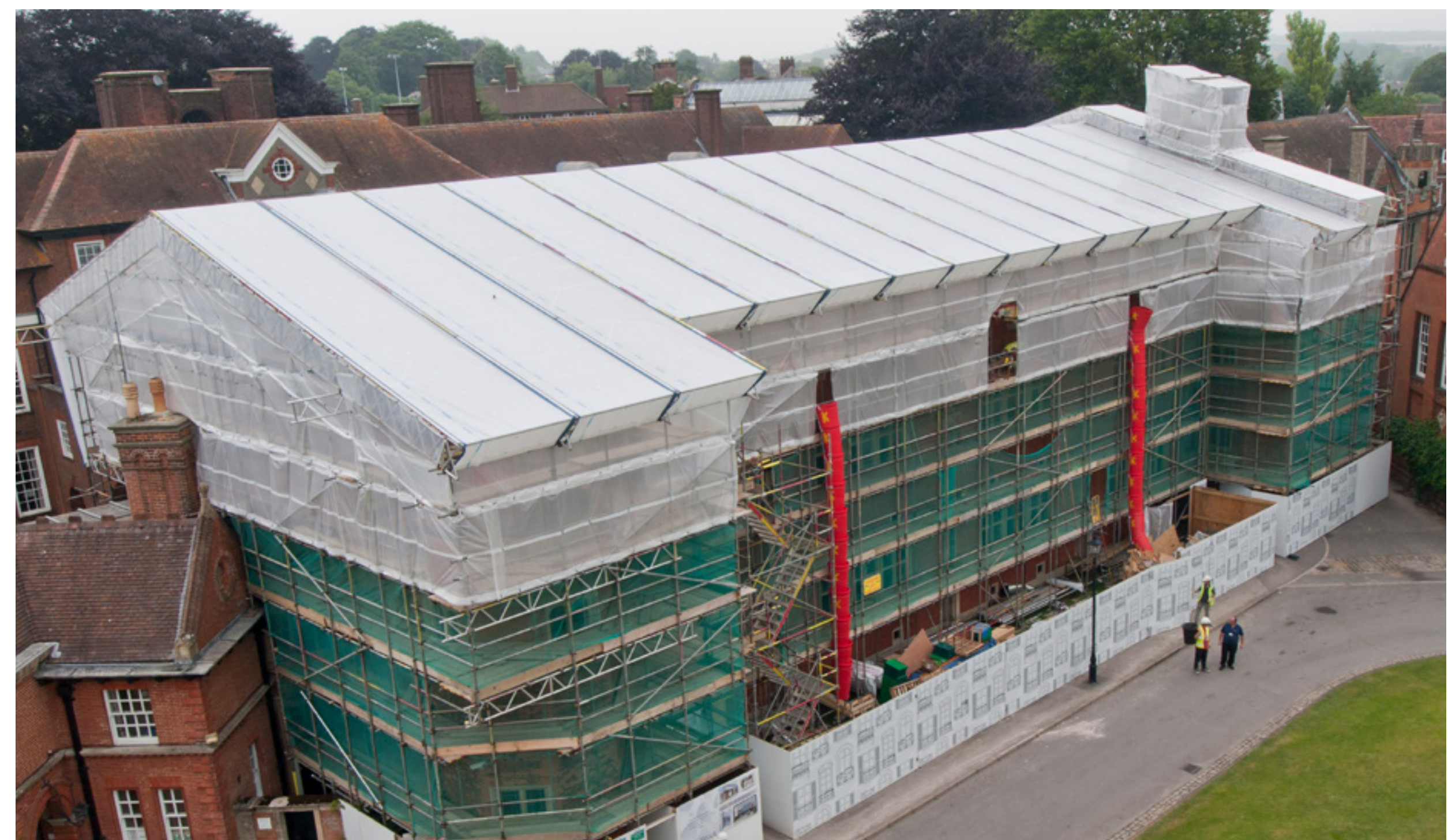
Marlborough College, Wiltshire: BMI Monarflex Temporary Roof Covering system
