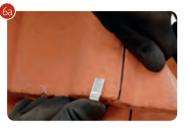
the tiles should not be more than 30mm from the hip batten. For Cambrian Slates: Each cut slate (for type see table below) must have at least two nails at the head and be clipped where possible. Continuous Hip itself acts as a third fixing.
