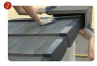
On gable end roofs, use left-hand and/ or right-hand Block-End Monoridge Tiles or Monoridge End Caps (LH/RH). Cut Monoridge Tiles should not be less than half their original length and should not be fixed within 450mm of the end of a ridge line. Carefully drill a 6mm diameter hole, 30mm in from the end of cut Monoridge Tiles. When using Cloaked Verge at the left-hand verge, cut a Profile Filler Unit to fill the open end.
