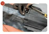
gaps at the eaves are covered. Remove the backing strip from the adhesive section and neatly dress onto the tiles. For optimal adhesion tiles should be clean and dry. Continue up the full length of the hip and over the ridge batten, overlapping each roll by at least 50mm.
