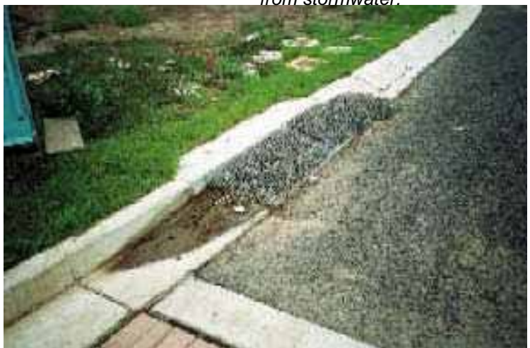
Photo 5: A Filter Fabric 'sausage' is very effective in settling coarse particles from stormwater.
