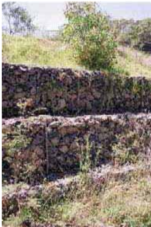
Photo 7: A benched embankment roadside cutting to minimise erosion.
