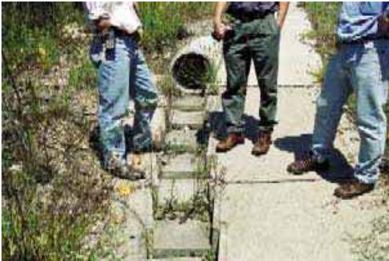
Photo 2: Sections of U-shaped concrete channel provide a safe delivery of roadside stormwater.
