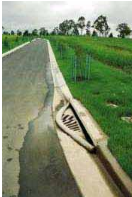
Photo 4: A Filter Fabric Drop Inlet Sediment Trap is both cost effective and efficient in keeping sediment out of stormwater systems.
