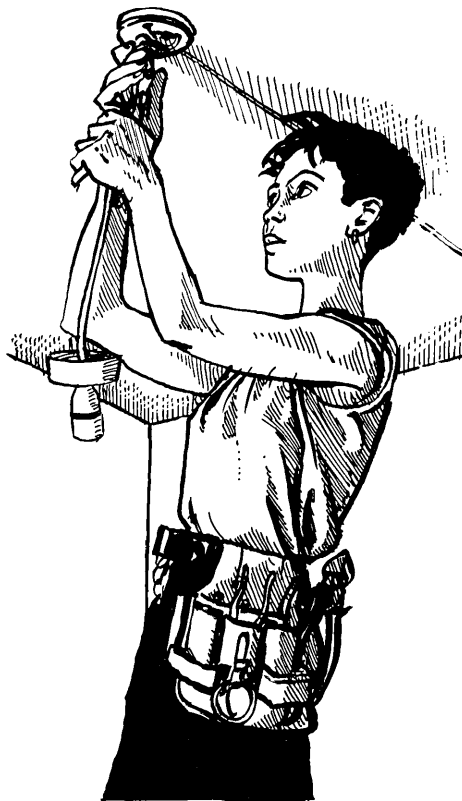
Wiring up a light socket.
