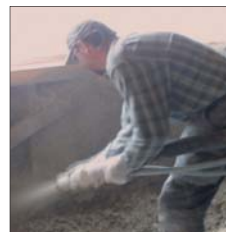
Hemp lime spray application
