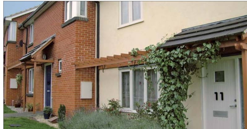
Suffolk Housing Association, Haverhill hempcrete house
