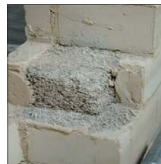
Hemp lime block wall
