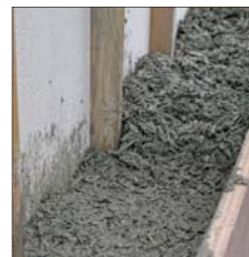
Hemp lime in shuttering
