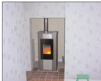
The automated wood pellet stove
