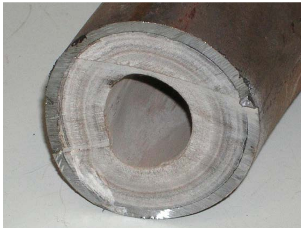
AN INDUSTRIAL PIPE THAT CARRIES WATER
