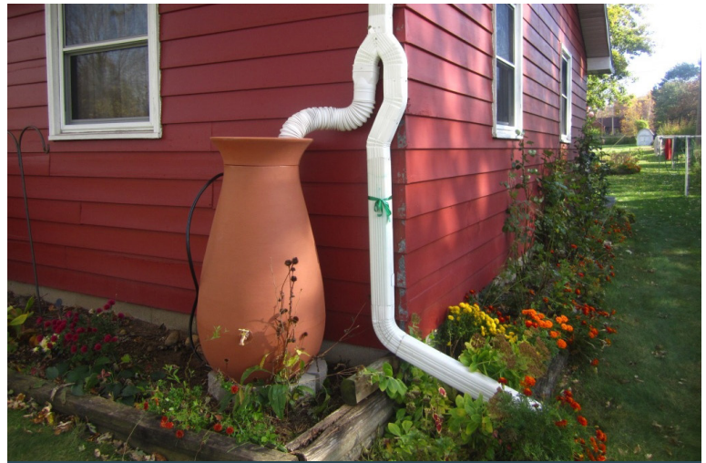
Gutters and Rain barrels channel and store roof runoff for later use. Spouts can also channel roof runoff to pervious areas such as lawns or to underground water storage such as cisterns.
