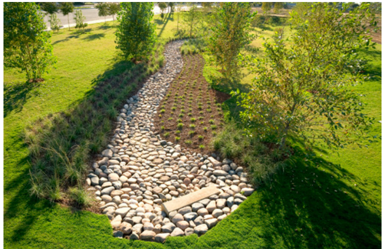
Infiltration trenches are one example of green infrastructure that helps reduce demand on drain pipes by retaining runoff.
