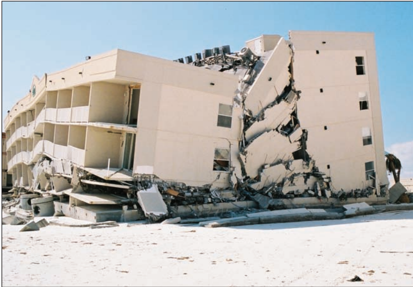
Figures 2-5 and 2-6. ORANGE BEACH, ALABAMA: Collapse of five-story, multi-family buildings on shallow foundations. (Source: FEMA 489)
