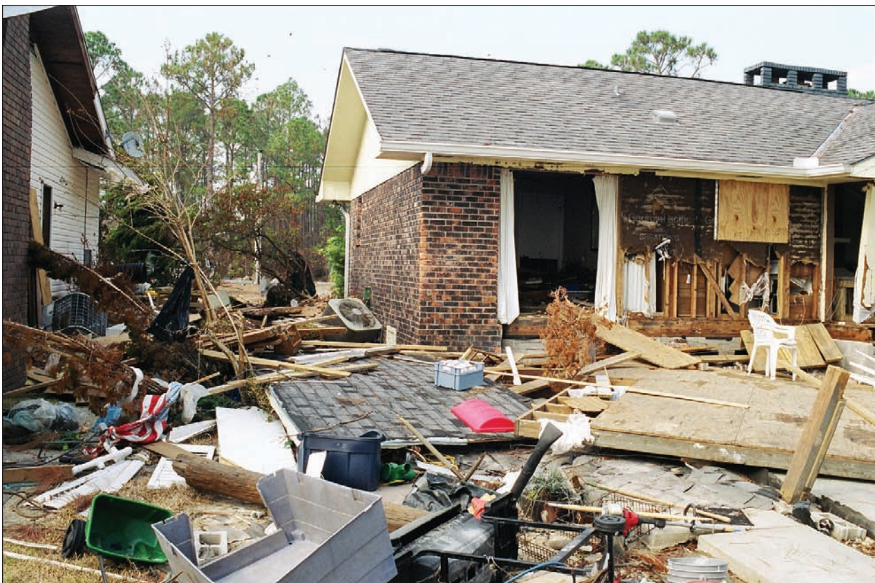
Figure 2-12. BIG LAGOON, ALABAMA: Buildings constructed on piles and elevated several feet above the base flood elevation (BFE) sustained less flood damage than adjacent buildings at lower elevations. (Source: FEMA 489)
