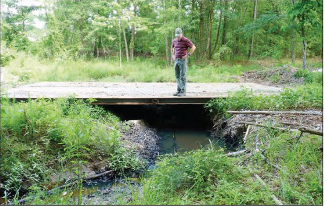
Installation of temporary bridges like this metal one can be used on temporary forest roads.
