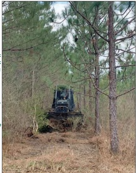
A bulldozer pushes a fireline.
