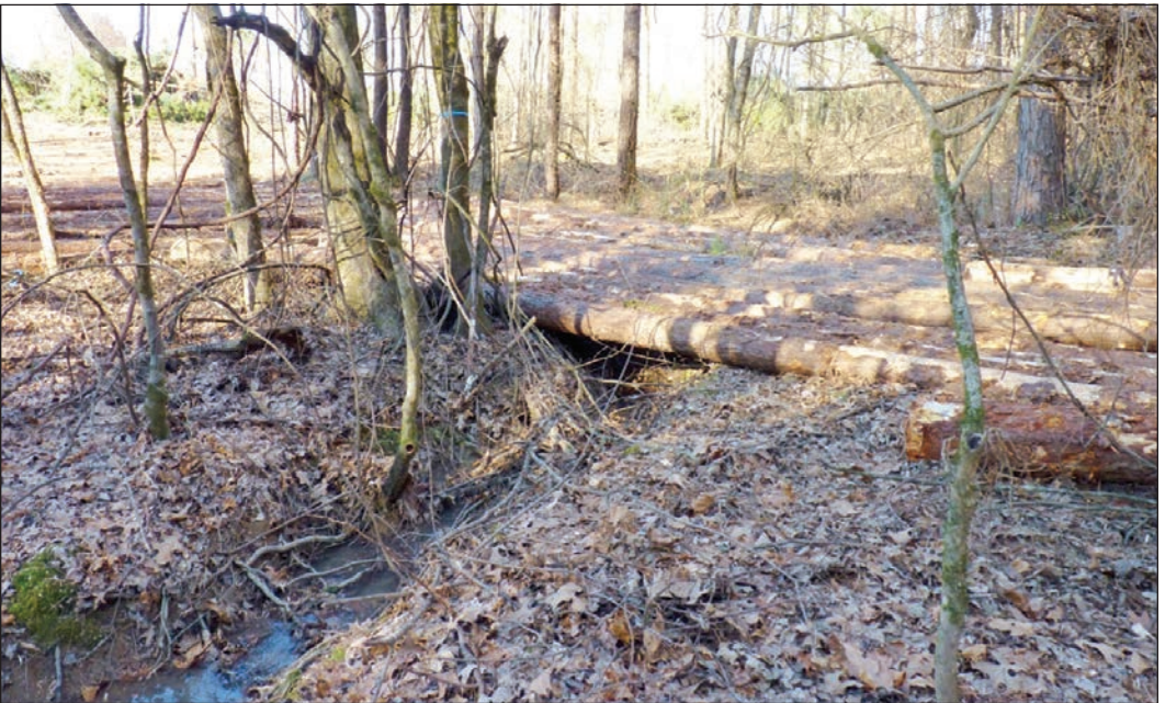
A log bridge is one way a temporary crossing can be made.
