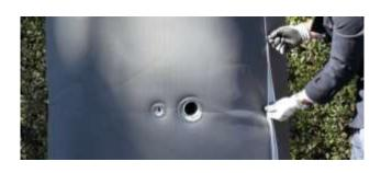
When the first panel is in place, fit the section to the left using the same process. Where the sections meet zip together. Make sure to relieve the stress from the zipper by pulling in the two sections either side of the zipper.
