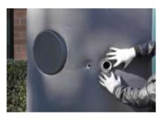
Line up the section that has the two larger holes with the flanges on the tank. The bottom of the insulation should be touching the ground. If there are further holes in the section fit them over the fittings ensuring the insulation is clear of the fittings.
