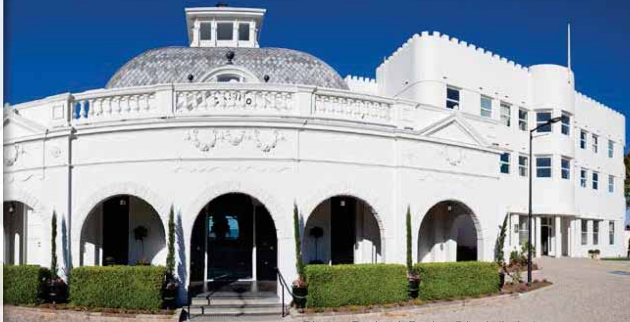
Rheem Tankpak Series 2 installed at Hydro Majestic Hotel - Blue Mountains, NSW
