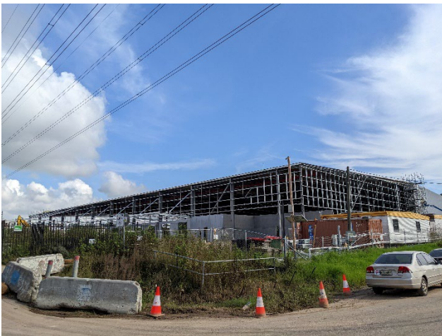
Picture 3 View of a new warehouse being constructed at 421-427 Flushcombe Road
