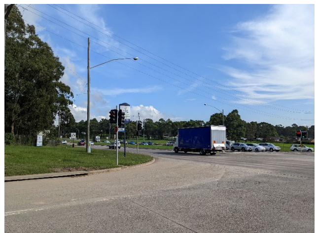
Picture 6 View of Great Western Highway looking north west
