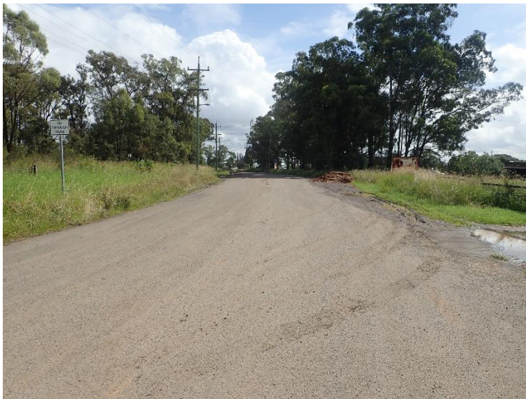
Figure 23. Yallock Place, looking north-west
