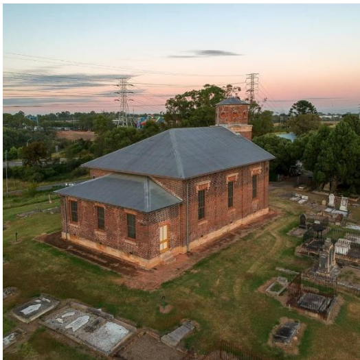
Figure 39. View to the south-west showing the dense mature vegetation to the west of St Bartholomew's
