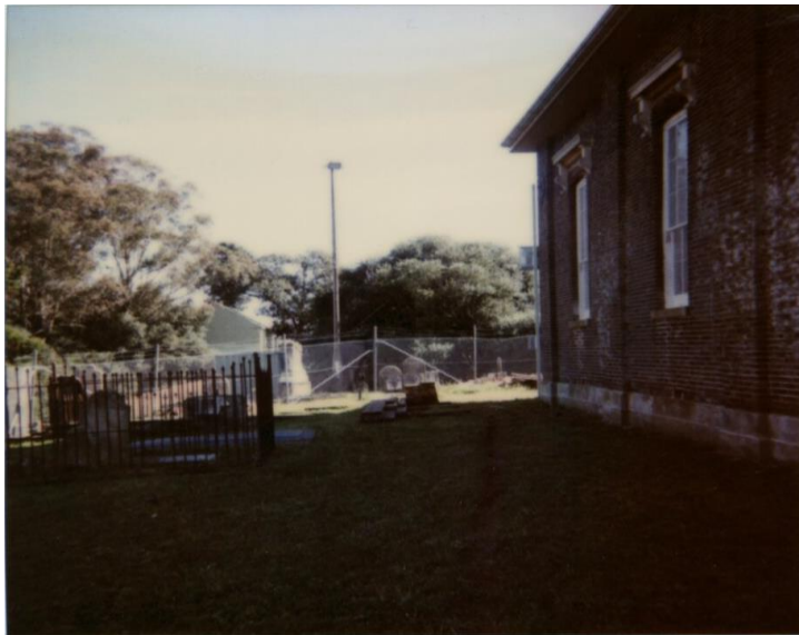
Figure 36. View along the side of St Bartholomew's Church facing west, 2000
