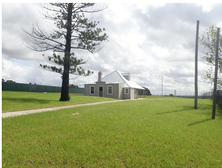
Figure 25. The rebuilt Former Police Residence / House, looking north-west
