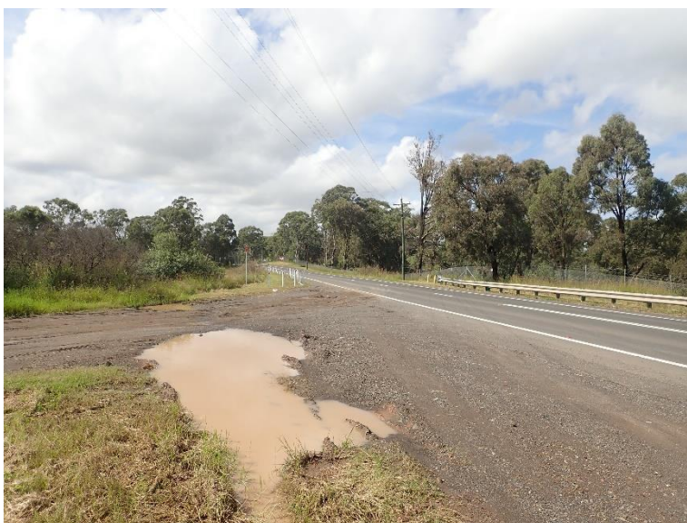
Figure 24. Reservoir Road, looking south-east
