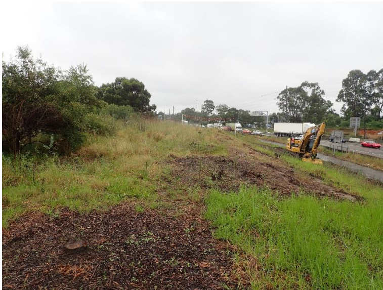
Figure 22. Works along Prospect Highway, looking south
