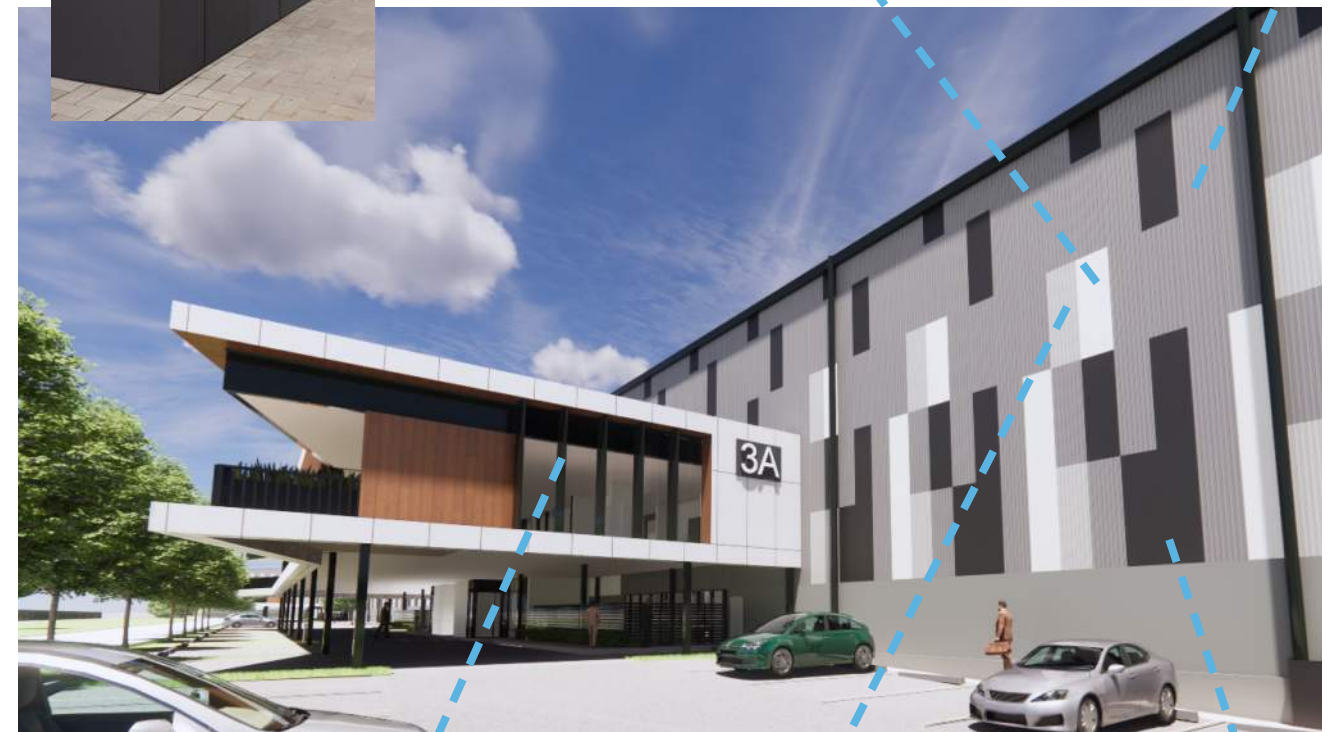
Figure: Warehouse & Office 3
