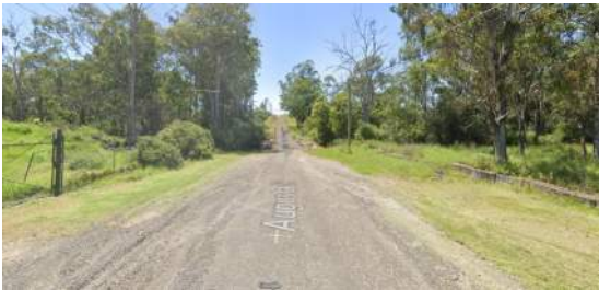
Augusta Street - Looking East
