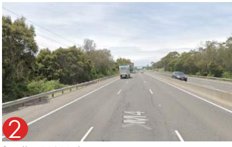
South - M4 Motorway
