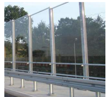
Polycarbonate Sound Barrier
