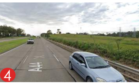
North - Great Western Highway
