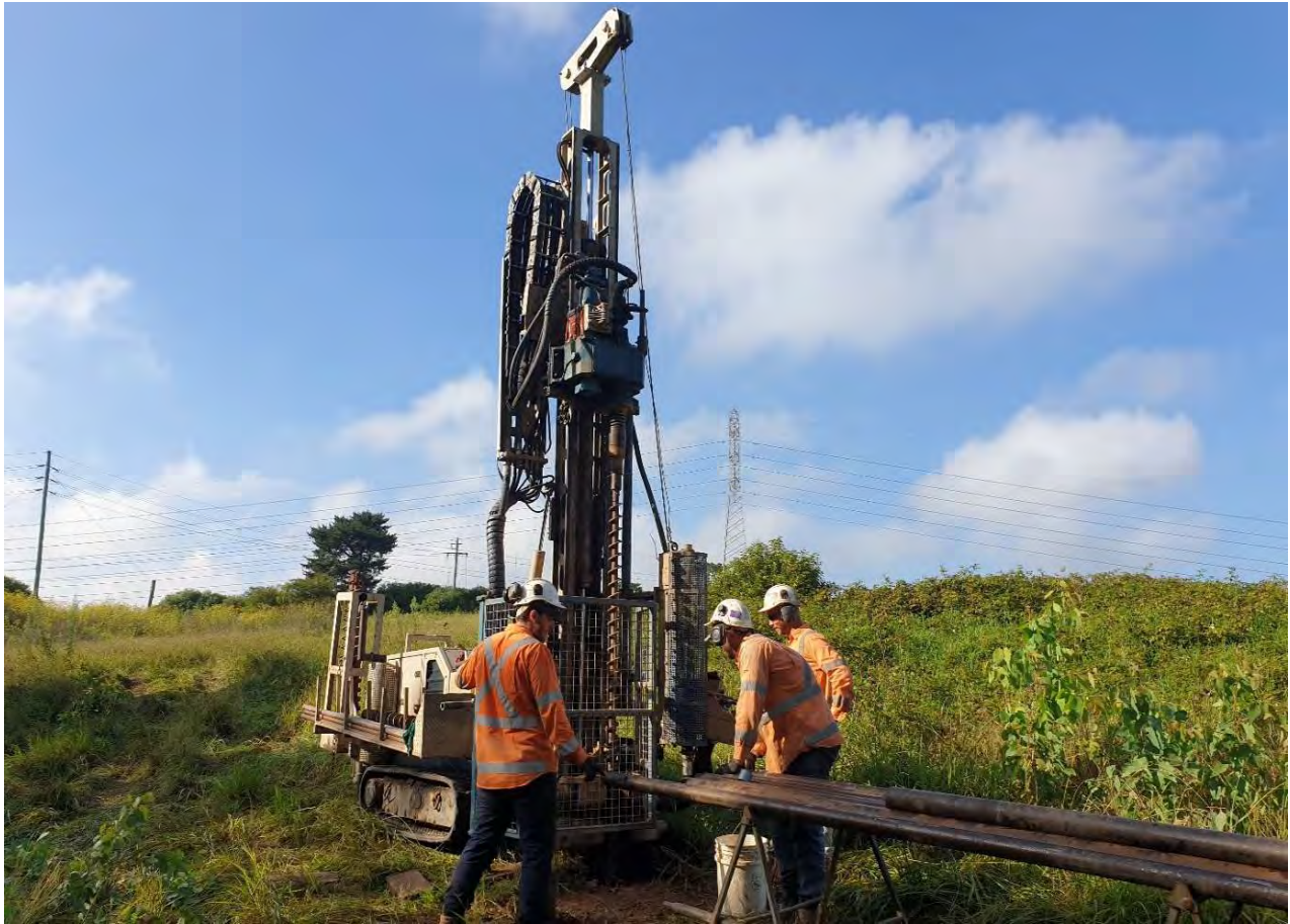
Photo 3 - Drill rig setup on BH12 (18/02/2022)
