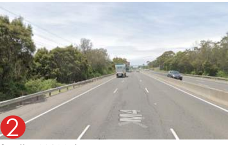
South - M4 Motorway
