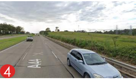
North - Great Western Highway
