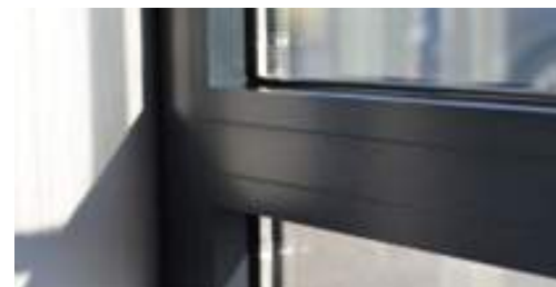
Black Powder Coated Framing to Glazing
