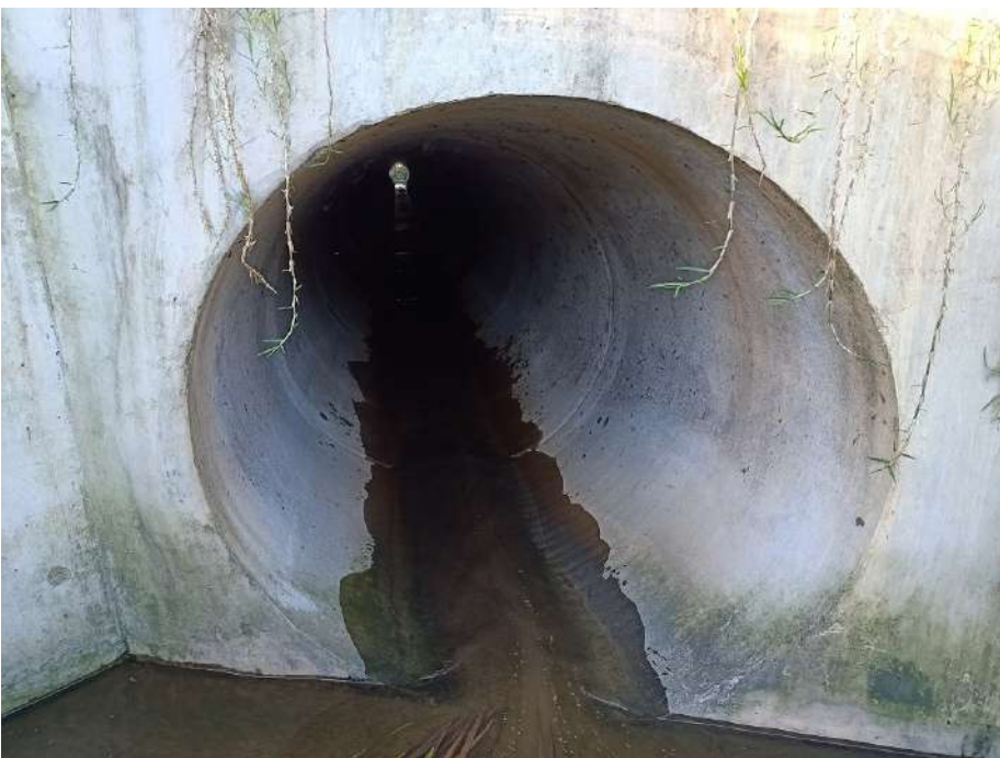
Plate 4. Culvert of Blacktown Creek with potential microbat roosting habitat
