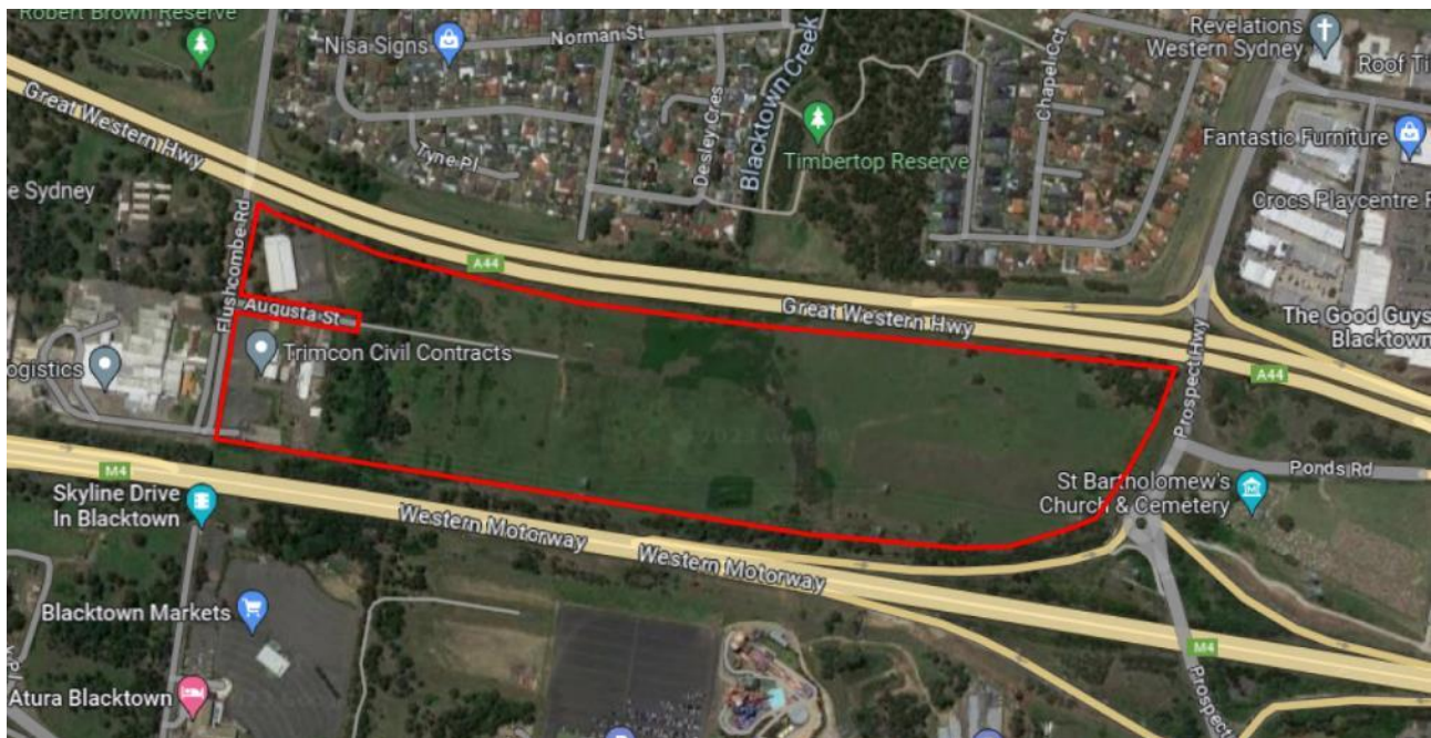
Figure 2-1: Aerial View of the Site (Source: google maps)
