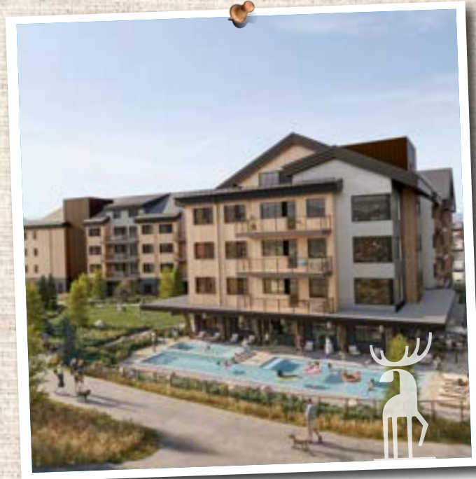
The Amble, our first residential community in Steamboat, will start construction in spring 2024, and we are working toward completing this 42-residence community on time and on budget.
