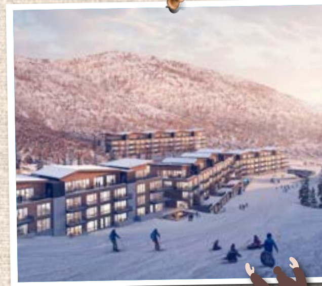
Founder's place Phase I is scheduled to be completed on time and on budget, with a projected completion by Q4 2024, when Phase II construction will start.
