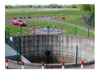
We operate a dedicated Flood & Pollution Control System across the site which is made up of four Total Organic Carbon (TOC) monitors and 10 polluted water holding tanks.
