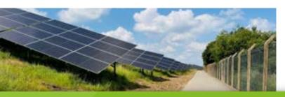
Installation of onsite renewable generation is a key component of our net zero journey. This year construction started on a 6.8-megawatt configuration of c. 12,000 solar PV panels on the 1.5km-long embankment know as the 'Alpha Bund', which provides residents of Marston green with protection from ground noise on the airfield.
