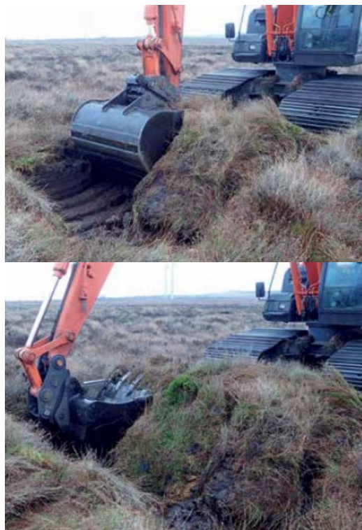
Figure 4 Creation of a wave dam (Short & Robson, 2016)
