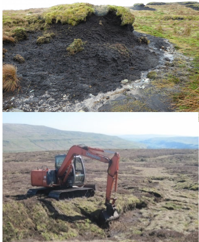
Figure 11 Top: Peat hagg. Bottom: Re-profiling of a hagg. Photo credit: Cumbria Wildlife Trust
