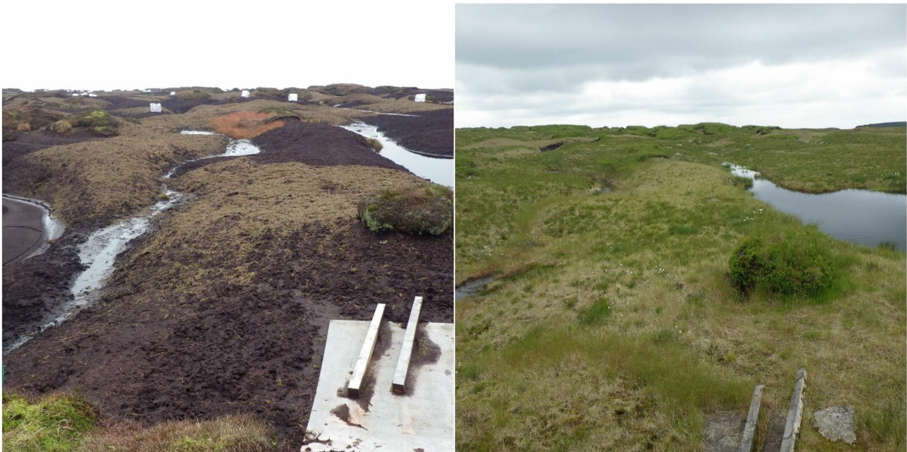
Figure 16 Bare peat restoration in the Peak District. Photo credit: Moors for the Future
