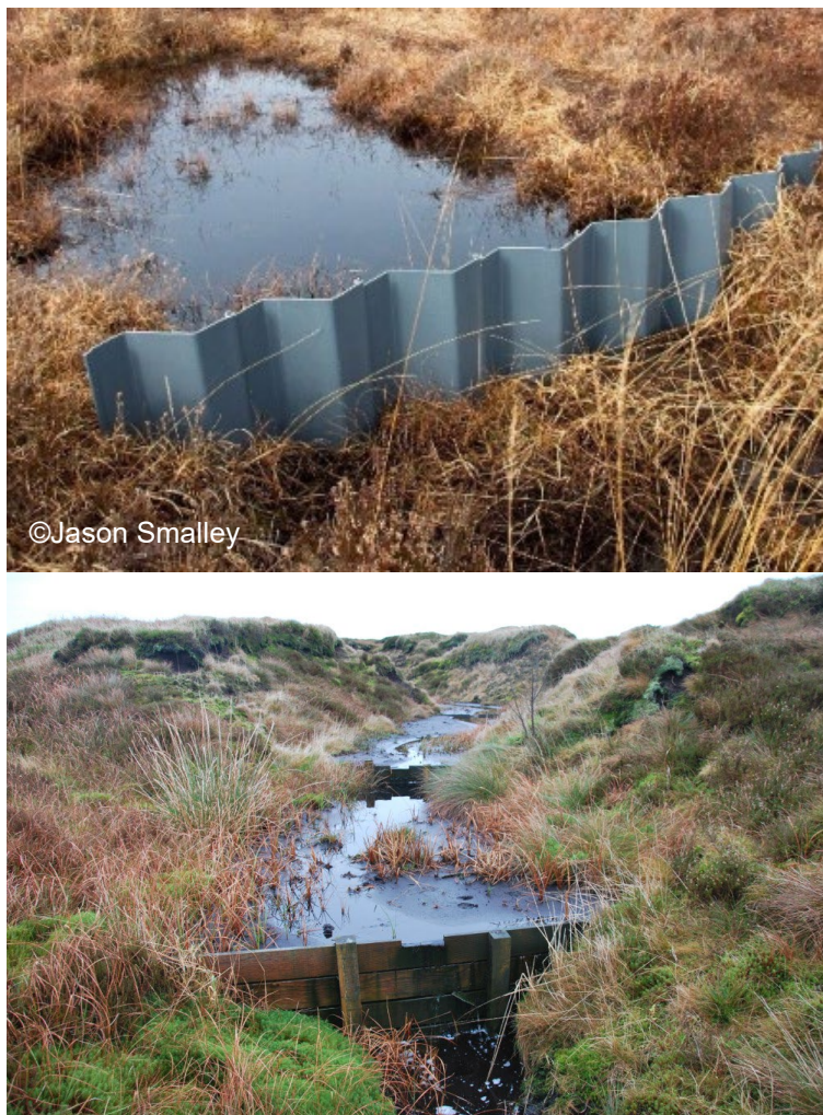
Figure 6 Top: Plastic piling in a raised bog (Thom, 2019); Bottom: Timber dams in a blanket bog gully. Photo credit: Moors for the Future
