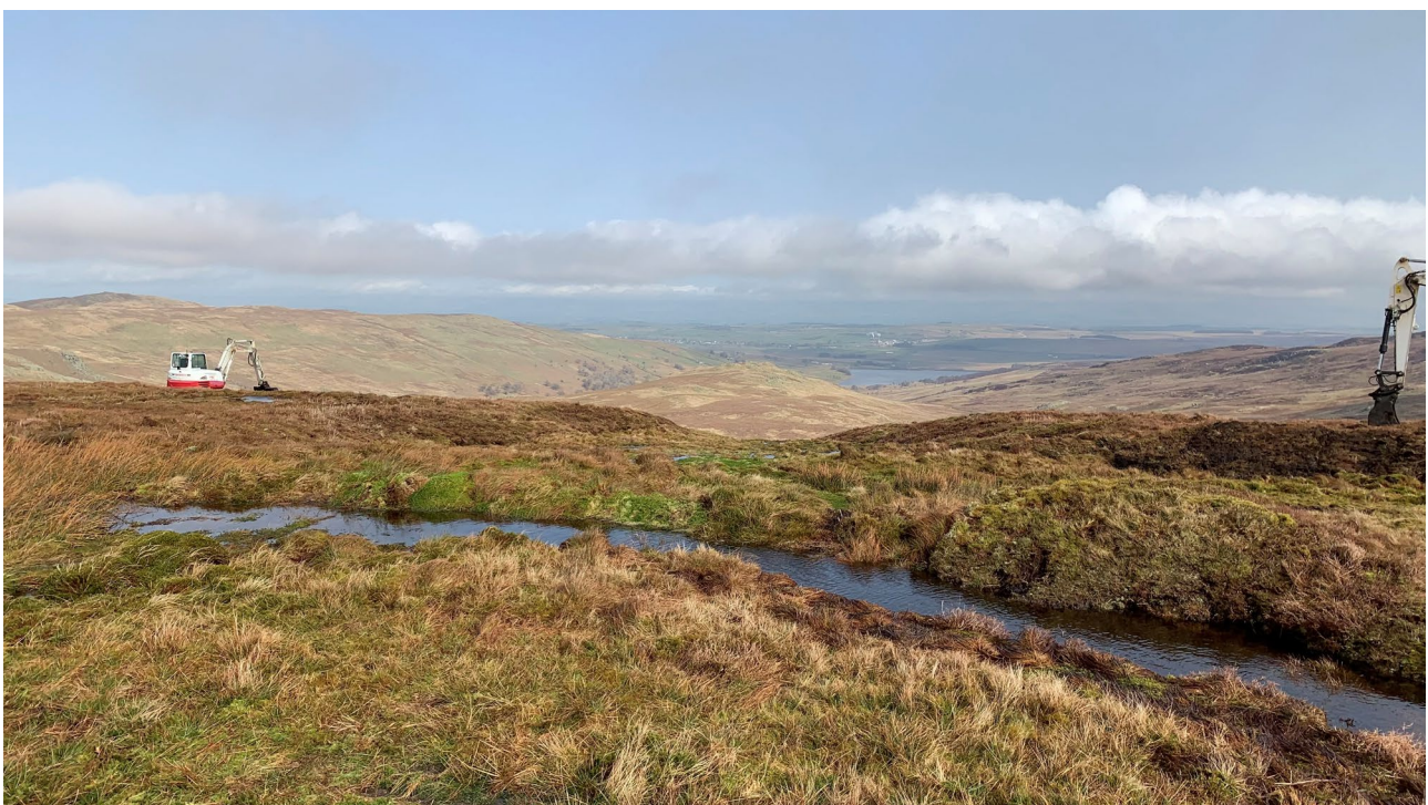
Figure 10 Newly created arc bund on degraded blanket peat constructed above a large erosion gully to slow the movement of water through the peat. Photo credit: Deborah Land
