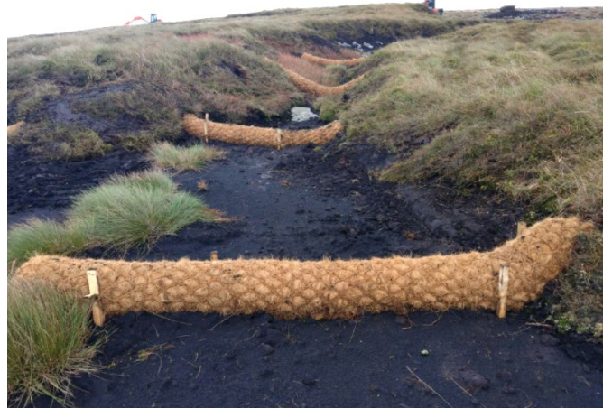
Figure 8 Top: Established heather bale dam (Photo credit: Moors for the Future). Bottom: Coir rolls on Pendle Hill, Lancashire. Photo credit: Conservfor Ltd
