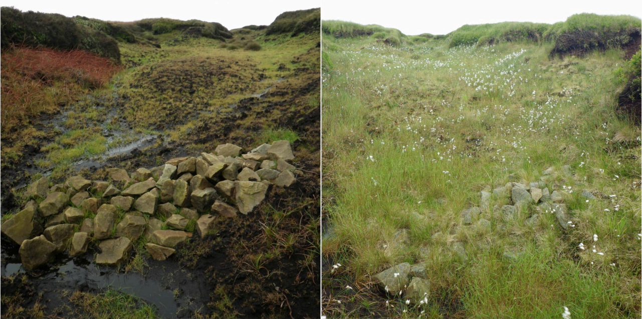
Figure 7 Stone dam installed in the Peak District. Photo Credit: Moors for the Future
