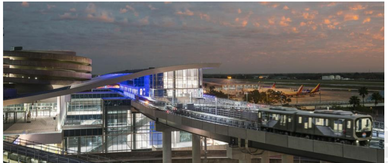
TPA ConRAC served by APM from Terminals. Photo courtesy of Arora Engineers
