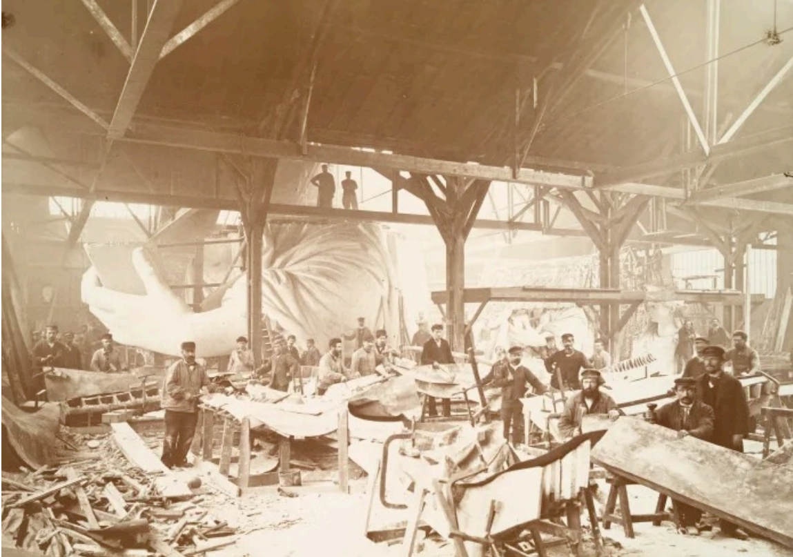
Men in a workshop hammering sheets of copper for the construction of the Statue of Liberty, circa 1883.
