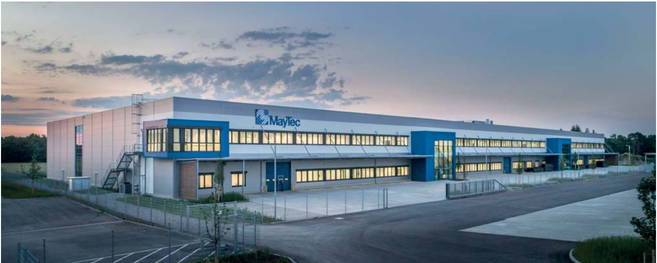
MayTec GmbH plant in Olching
