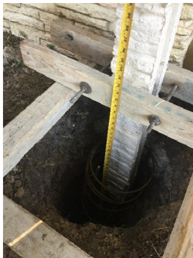
Figure 6: Post to Foundation
