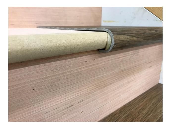
Riser material should be cut net to fit between the SimpleStair treads.
