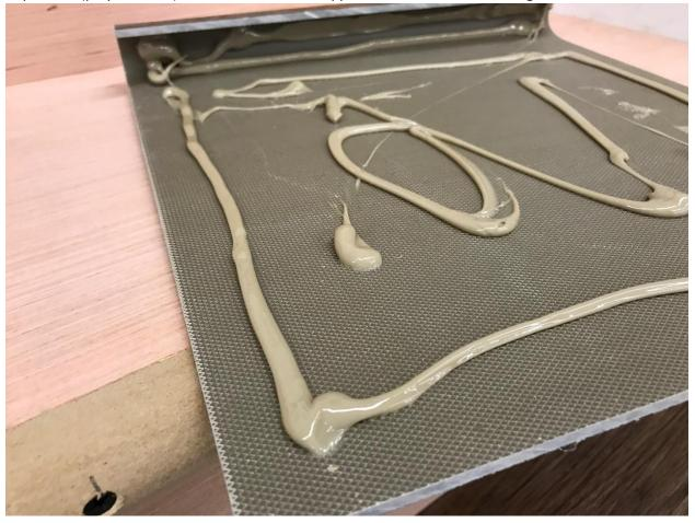
Triple Stick (polyurethane) adhesive needs to be applied inside the curved nosing.
