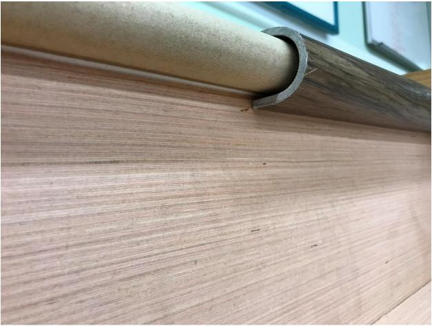
Underside of the SimpleStair curve may need to be cut back to create a tighter fit.
