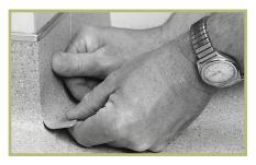
Check the fill piece for accurate fit. Make any minor adjustments to the plug as necessary to fill the space correctly. Remove the fitted fill piece and apply the appropriate adhesive. Reposition the fill piece and apply seam sealer
