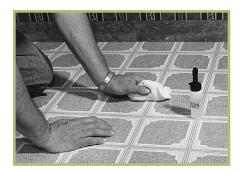
Before sealing the seam, make sure the seam cut is clean, dry, and free of adhesive contamination. Shake the seam sealer container to blend the ingredients and allow air bubbles to disperse (usually 15 minutes) before pouring sealer into the applicator bottle. Fill the bottle at least 2/3 full with the appropriate seam sealer and tightly screw on the VST applicator tip.
