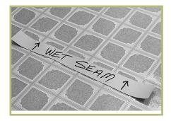
You must apply seam sealer into the seam cut and leave a bead of sealer approximately 1/8" wide centered on the seam. This applies to all Mannington Residential products. To avoid walking on the seam, mark it with a scrap piece of floor covering.
