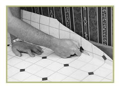
Using a sharp knife held parallel to the wall, trim away the excess material until the product is flat on the floor. Hold your cutting hand so the palm faces the wall and is out in front of you within your comfort zone. Ride the knife point at the juncture of the floor and the wall. Make sure the knife blade is flexible enough to allow some pressure to be applied to it. Hook knives and Ward type knives work well, but utility and Airway type knives do not.
