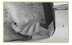
Scribe and cut the outside corners of the felt using a utility knife.
