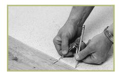
Slide the flashing sheet away from the wall (Wall A) until it lies flat on the floor and against the wall. Go back to the key mark you made on the resilient and subfloor and you will notice the mark is no longer in alignment. Set your bar scriber or dividers to that difference.
