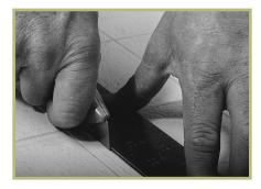
With the sheets aligned, position the steel straightedge so it completely covers the grout line of the top sheet. Using the straightedge as a guide, cut the length of the seam in the "shadow" of the grout line with a utility knife. This technique will ensure that all grout lines are of the same width. This is important, since you will completely cut away the bottom sheet grout line and will leave the grout line of the top sheet intact.
