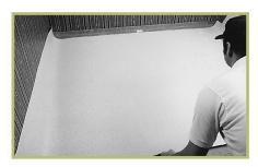
Slide the resilient flooring to the wall. The sheet should now be positioned on the 6" reference line and next to the long wall.
