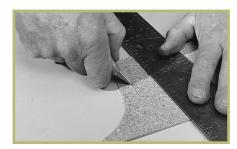
Cut along the scribed line at a 45° angle with a curved trim knife or a utility blade while holding the plug steady with a metal ruler and your other hand. When cutting, leave the face of the plug longer than the back.
