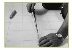
Once the seam is cut, remove the selvage edge and turn back the material to expose the subfloor.
