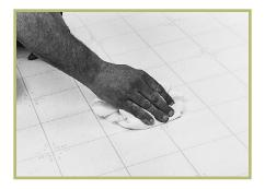
Thoroughly clean the seam area with a clean white cloth and wipe dry. Remove any adhesive that has dried on the surface with a clean white cloth dampened with a good quality-grade mineral spirits or painter's naphtha. Avoid wiping down or across the seam cut with a soiled cloth. Keep the seam cut free of soil, adhesives, or contaminants.
