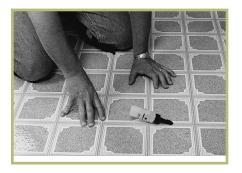
Seam sealer flow will stop when hand pressure is removed. This allows you to leave the applicator inserted in the seam cut when you reposition yourself along the length of the seam. This helps eliminate the chance of sealer skips caused by repositioning the applicator during seaming.
