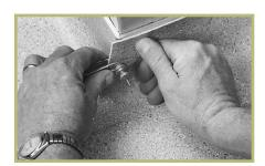
The most demanding aspect of a coved installation is forming the outside corners. Fill outside corners with a boot-type plug, rather than a V-type plug, on the least visible wall. The plugged corner fill piece should extend back at least several inches from the corner. The seam of the floor should be below the cove stick. Using an underscriber, scribe the back of the plug at the corner. This will mark the pattern of the corner on the plug.
