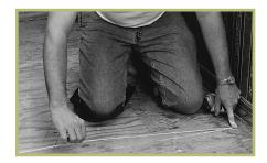
When installing 6' wide resilient flooring, snap a chalk line 6" off the wall. Also, make two additional reference marks in the center of that area. Snap a chalk line marking the center of the sheet on the floor and mark that same distance with a piece of tape on the wall.
