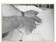
Cut a "V" when making inside relief cuts. Use your left hand to find the corner with your thumb and forefinger. Place them over floor covering into corner about 2" up the wall. Make outside relief cuts with the floor covering held back from the corner. Cut the material from the face
