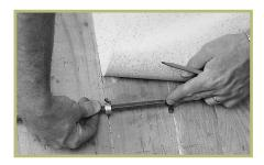
Position material squarely in room with about 2" flashed up each end of wall. Material should be positioned against the long wall overlapping the 6" reference line. Trace the edge of the sheet with a pencil marking onto the subfloor. Set dividers, or bar scriber if you need to transcribe deeper offsets, to the distance between the edge of material (pencil mark) and reference line.
