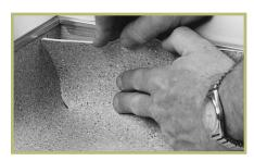
Dry fit the material. Inside corners should fit snugly, but not be forced into position. Make sure to always position the shorter side first and then the longer side. Gently pull the material away from the wall.
