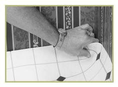
Make inside and outside corner relief cuts before trimming walls. When making any relief cuts, make them all to one side of the room first. If you need to shift floor covering, you can shift it into the cuts. If you make relief cuts on both sides of the room, when you shift the floor covering you will be short of material on one side or the other.
