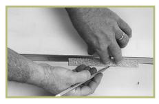
Tack the scribing felt to the wall with brad type nails before you begin to scribe it. Use a combination square, a small metal ruler, or a 1" piece of resilient to pattern scribe the felt. Fit the scribing tool up inside the cove cap and scribe the felt by sliding the tool along the cap as you mark the felt with a pencil.
