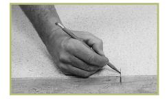
Now fit the two remaining walls, which we will name Wall A and Wall B. Make a reference mark (key mark) at the edge of the resilient sheet extending onto the subfloor with a pencil. Place a piece of tape on the long wall (the opposite edge of the sheet), visually aligning it to the pencil mark you just made on the resilient and subfloor. You will now have a reference mark on the right side of the sheet and a reference mark on the left side.
