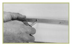
Measure desired height for the cove caps at each corner and strike a chalk line. Attach aluminum or vinyl cove caps at this height using flathead nails with a hammer or brad pusher, or use contact cement. Always miter inside and outside corners in the cap. When mitering the outside corners, file the ends of the cap smooth. You can use a specially designed miter tool with interchangeable die sets to make corners on the cove cap. This tool eliminates sharp edges at the outside corners.
