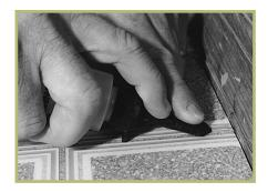
Check the flow of sealer through the applicator tip on a scrap piece of material before use. If the flow is restricted, insert the cleaning wire into the tip to clear the obstruction. Insert the plastic fin of the VST slightly back from one end of the wall and push forward to make full penetration of the fin. Use your forefinger to apply a downward pressure on the flat, textured "head" of the VST.
