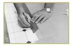
Using the same roofing square or dividers, transfer the marks on the pattern to the sheet goods, making a perfect duplicate of the floor. Be sure to keep the dividers set to the same measurement you started with and use the same leg of the square you used to make the pattern. To ensure correct pattern transfer, the person who performed the pattern scribing should also transfer the pattern onto the resilient flooring.
