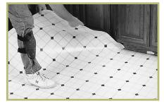
Now that the transfer and cutout are complete, the material is ready to be installed. The floor covering is an exact duplicate of the floor, with all excess material removed and all cuts made for possible obstacles. Place the material into the room and fasten as required.
