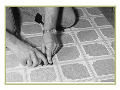
Gently squeeze the bottle to start the flow of the sealer. In a slow, continuous motion, pull the applicator along the length of the seam. The correct angle of the applicator tip to the seam is determined by the flat support or "landing face" of the VST. Most importantly, once the tip is inserted into the seam cut, it does not need to be removed until the seam is sealed, ensuring complete sealer application along the entire length of the seam.
