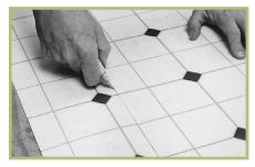
Follow the pencil marks on the surface of the resilient with a knife or scissors. Use caution so you don't damage the underfloor you're working over. A hookblade utility knife may make this easier.
