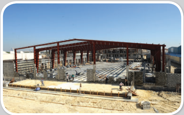
Aerial view of the multi-purpose hall
