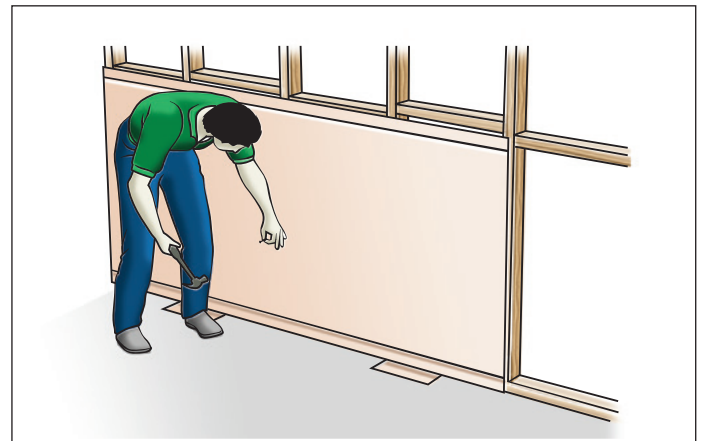
FIGURE 4 FIXING FIRST SHEET
