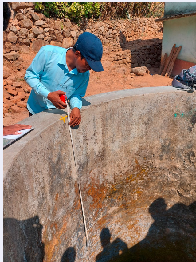
Photo: Community resource person “Jal Bandhu” at the Gram Vikas project site monitoring the water level in a well. © Neha Bhadbhade, SOPPECOM
