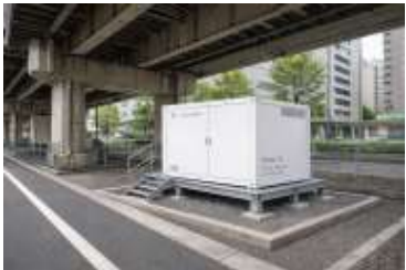
Areas under elevated tracks
