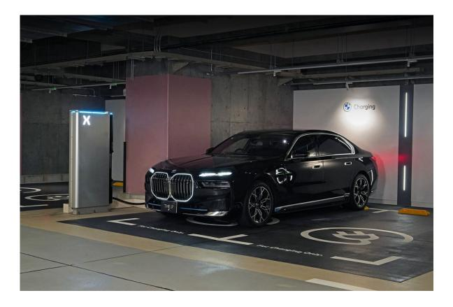
This charging station will be accessible to all electric vehicle owners, not just BMW and MINI drivers. Users can reserve charging sessions via the PowerX App, ensuring a seamless and wait-free experience. The installed chargers support ultrafast charging with a maximum output of 150kW, making them among the fastest in Japan. Users can charge for up to 60 minutes, allowing them to enjoy the shops, restaurants, and cafes at Azabudai Hills while their vehicles charge.
