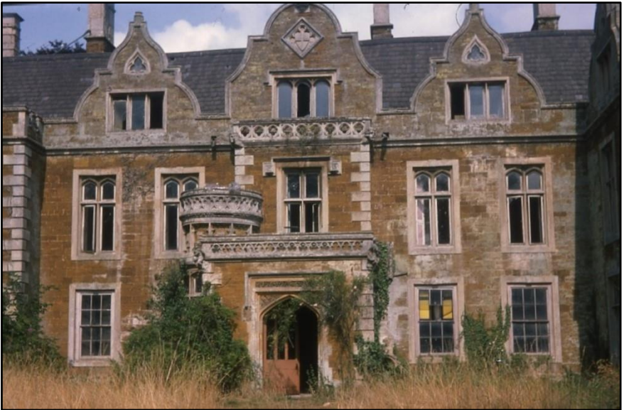
The south entrance, prior to the total renovation of the Hall, early 1970s From a collection of photographs donated by Ted Amey.
