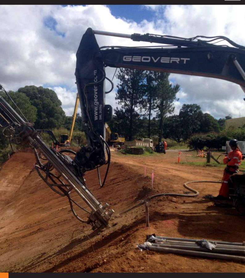
MILLAA MILLAA-MALANDA ROAD SLOPE STABILISATION SOIL NAIL SLOPE STABILISATION WITH ACTIVE MESH
