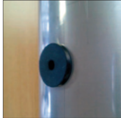
Fig. 2: Installation of Flue Sensor Mounting Plug
